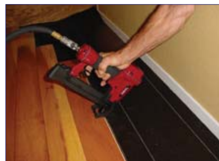
Using the dual trigger to fasten, with a reverse grip if needed in tight quarters.
